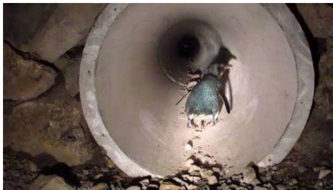
Figure B.8 Little penguins using an underpass installed to allow access to nesting habitat without crossing the road (reprinted from Dunlop, 2016)
